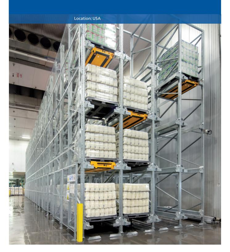
Dairy products supplier and distributor Producers Dairy recently installed a semi-automated Pallet Shuttle for its 50,000 ft<sup>2</sup> cooler at its plant in Fresno, California. The Pallet Shuttle replaced the company's outdated and inoperable pallet racking system. By installing the Pallet Shuttle system, the firm was able to double its capacity and prepare 300 orders per day.
