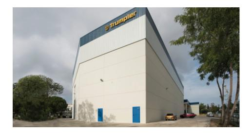
site's design was based on the dimensions of the automated warehouse to make full use of the available space, i.e., the racks were designed first and then the building was constructed. Thus, Trumpler obtained a 2,512 pallet storage capacity for raw materials and finished products.
