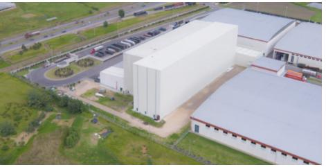
Grupo Familia, a company specializing in personal care and hygiene products, has a 115' high automated clad-rack warehouse capable of handling around 17,000 pallets. In the supply of the warehouse, located in the Colombian municipality of Cajicá, Mecalux has also included the Easy WMS warehouse management system and the Galileo control program, which are tasked with monitoring and executing the movements related to the logistics process.
