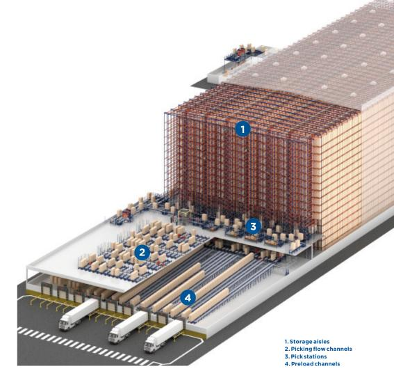
To maintain a continuous flow of movements, a 20-foot-high raised tunnel connects the outputs from the chocolate and cookie production lines directly to the warehouse. Inside the tunnel, an automatic conveyor line runs along the side of the logistics complex, extending the front of the rack-supported building. Thanks to the conveyor's accumulation capacity, the pallets can remain on stand-by temporarily, awaiting entry in an orderly manner and without needing to be placed on the floor.
